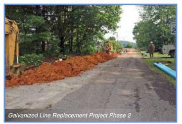
The replacement of WCSA's galvanized piping has been accompanied by a great deal of planning for the future. Lines are sized to meet the needs of customers 40 or more years down the road. In addition, galvanized line could not provide fire flow, and the majority of the new lines being installed include new fire hydrants. Since January 2010, WCSA has increased the number of fire hydrants from 1,076 to 1,616.
