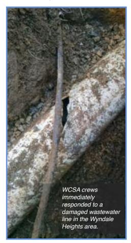
streets, presenting an additional challenge of avoiding damage to private property when parking off the road to keep from blocking traffic. The crew spots a busted line that has broken in a low spot. The resulting break is allowing rainwater to drain into the wastewater system. The crew sets up their equipment and begins digging.
