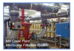
membranes that protect potable water supplies are at the heart of any system. They require constant monitoring and care to operate properly. In this instance, because of the heavy burden of particulate that reached the plant, all three skids of membranes were stretched and, in some cases, ruptured."
