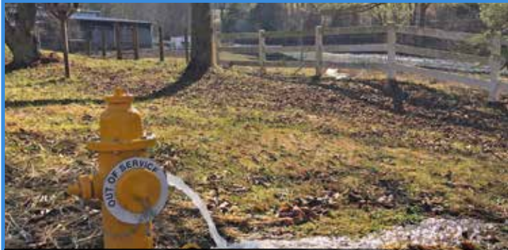
Line flushing to prepare for water quality testing at site of recently completed Rich Valley Road Water Line Extension Project
