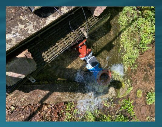
Cole Spring – Overflow Meter installed 4-inch Mag Meter
